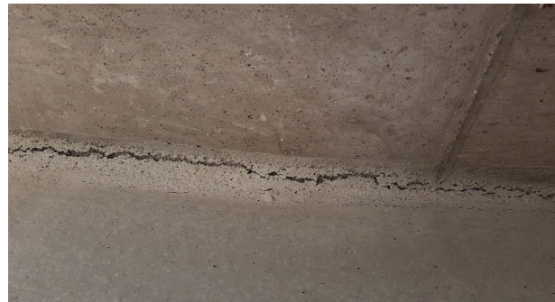
b) Flooring work
