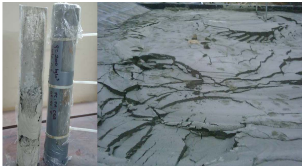
a) Light weight filling work
