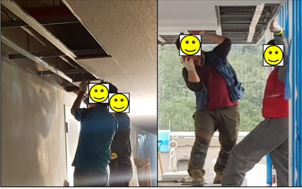
Fig. 2. Worker with no safety helmets
