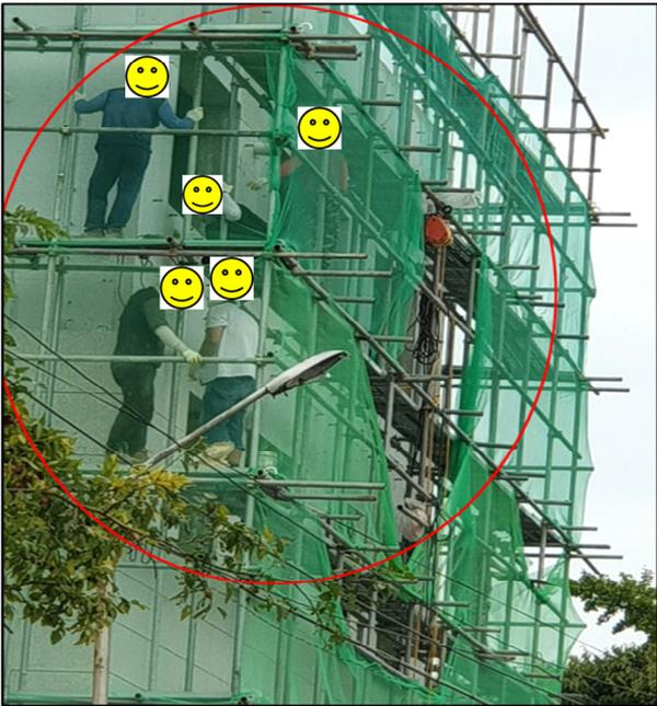
Fig. 3. Worker without protective equipment
