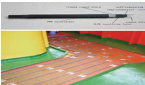
Fig. 1 Deck walk-way with heating cable
