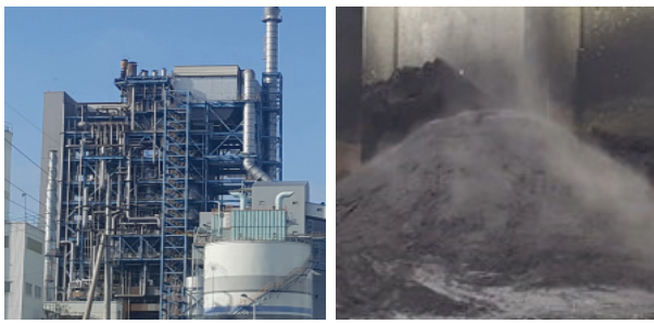
(a) Facility view (b) Slag occurrence Fig. 1. Integrated Gasification Combined Cycle(IGCC)
