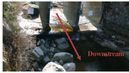
(b) Concrete box structures of uyidong valley
