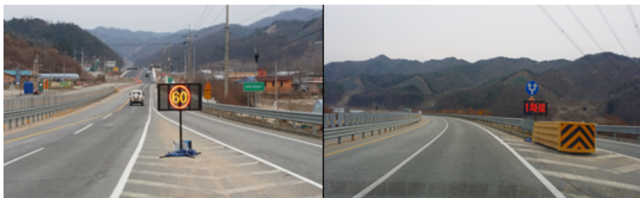
<Fig. 3> PVMS employed in 200m and 500m upstream of the work zone
