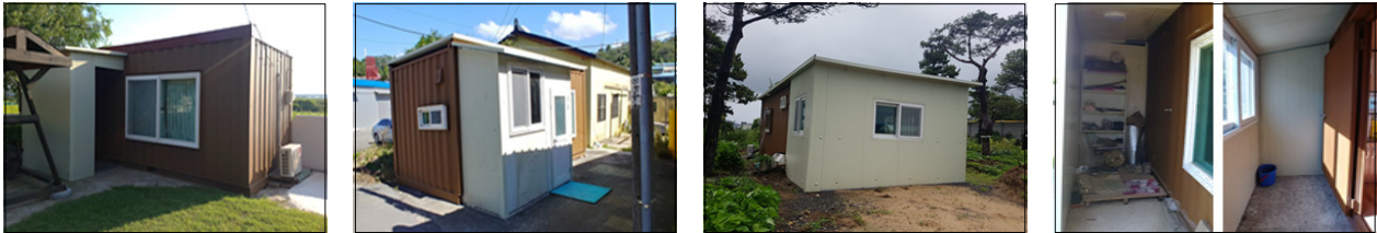
Fig. 2. Construction of additional entrance to Residential container
