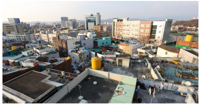
(d) Possible fire transfer due to adjacent buildings
