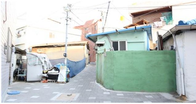
(a) Possible of collapse due to old residential facilities
