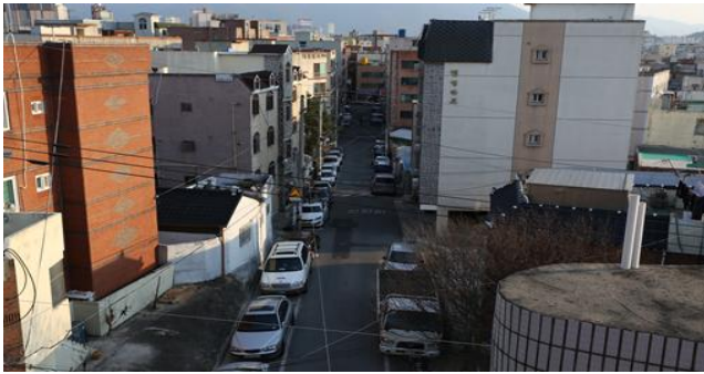
(c) Unable to enter fire truck due to narrow parking space
