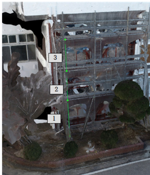
Fig. 7. Measurement of Wale Distance of Scaffold
