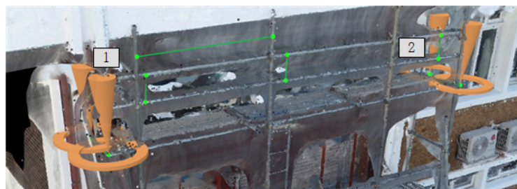
Fig. 5. Measurement of Beam Distance of Scaffold
