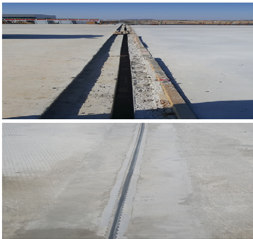
Fig. 2. Steel monocell expansion joint installed on the site
