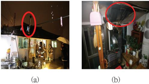
Fig. 3 (a) View of the building and installation of exhaust system on roof (b) Charred ceiling by radiant heat
