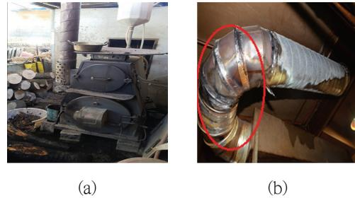
Fig. 4 (a) Wood stove in a fire place (b) Charred exhaust system
