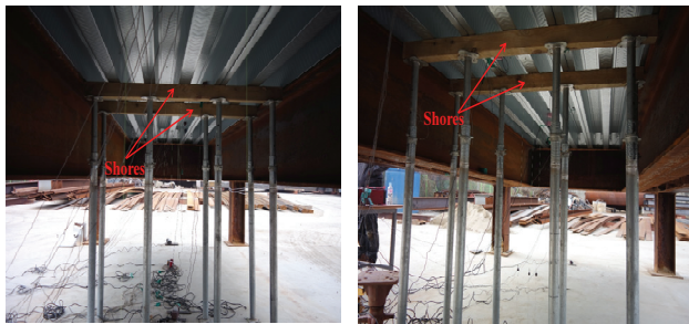
Fig. 6 Location of supports and shape of filler
