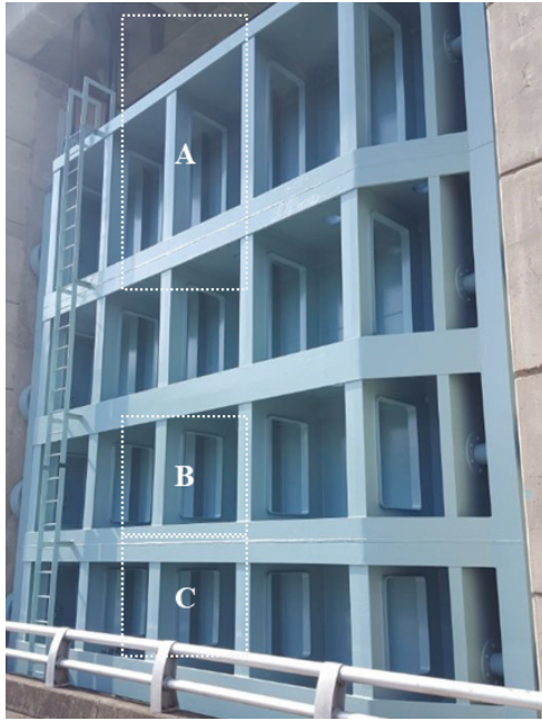
Fig. 2 Monitoring floor for a target steel water gate
