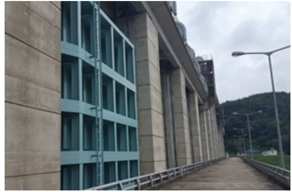
Fig. 1 Target steel water gate
