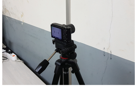
Fig. 4 Maximum Crack Width Test Set-Up
