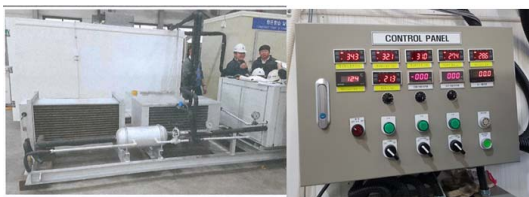
Fig. 8. Experiment of Heat Exchanger Using CO 2 Natural Refrigerant.
