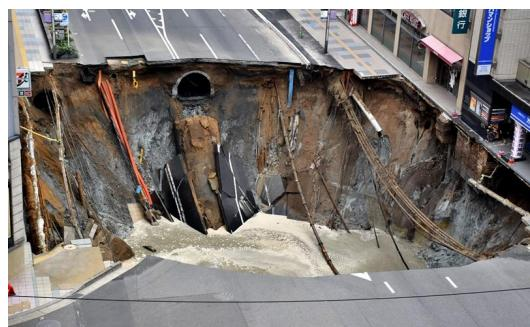
Fig. 1. Subsidence and sink hole in road
