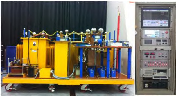
Figure 8. Impulse current generation system.
