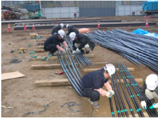
Fig. 4. Manjet tube and U-GIP injection pipe
