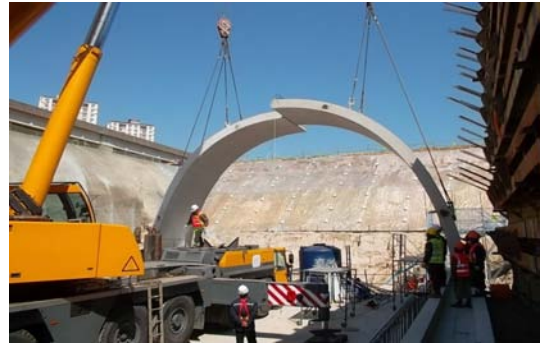
(b) Erection of the first two segments
