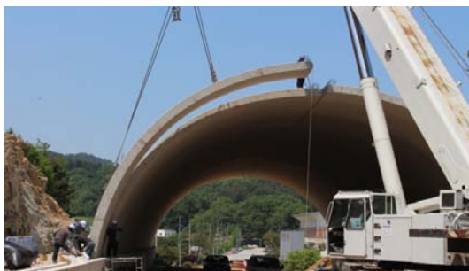
(a) During construction
