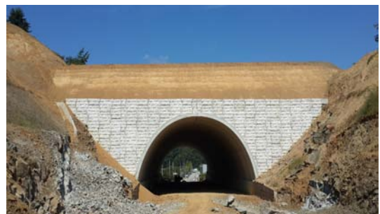
(b) After construction
