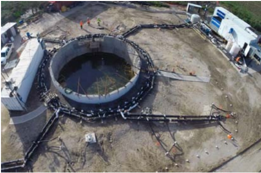
(a) Launching shaft for earth pressure balanced (EPB) TBM (Shawn et al., 2016)
