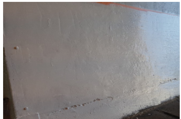
(f) Insulation construction completed (2)
