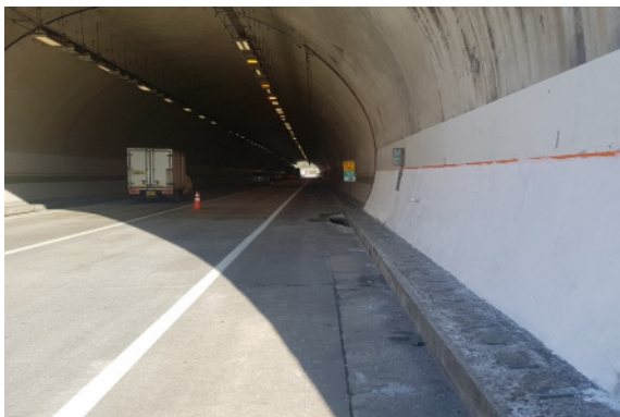
(e) Insulation construction completed (1)
