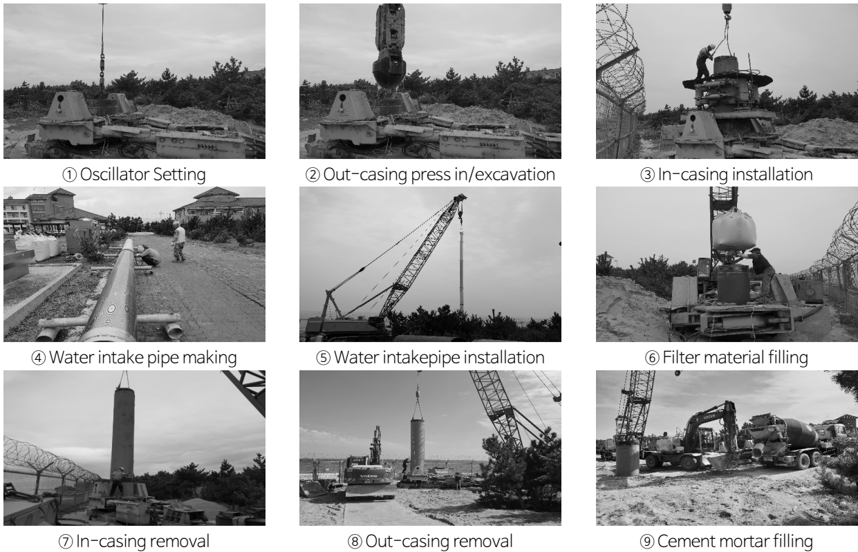
Fig. 3. Photograph of installation process(SD1200(A)).
