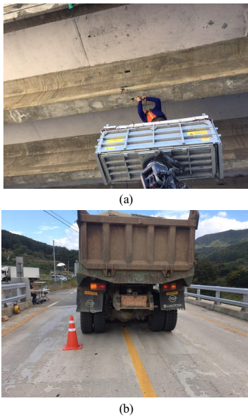
Fig. 2. Vehicle loading test (a) installation of sensors (b) static loading test
