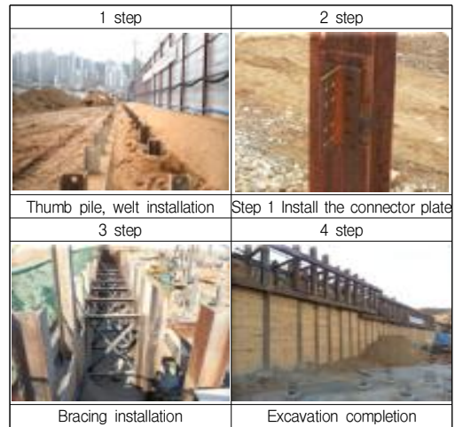
Fig. 5. Test construction flow chart
