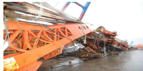
(b) Fractured and deformed state of the leader & the backstay (Kim et al., 2014)
