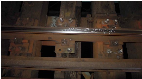
(b) 부식(Corrosion)
