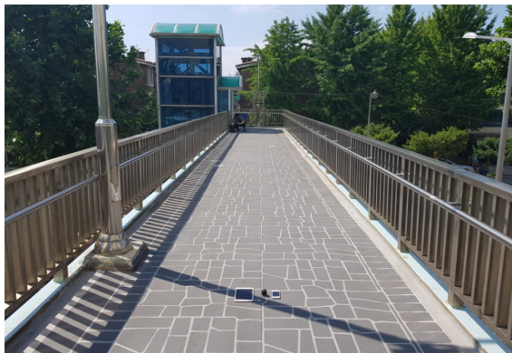
<Fig. 2> Footbridge (S-1)
