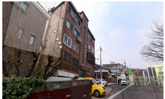
Fig. 7. Example of result difference (2) Existing(steep land) → Testing(mild land)
