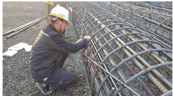
(b) Load transfer sensor installation
