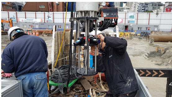
(a) System installation
