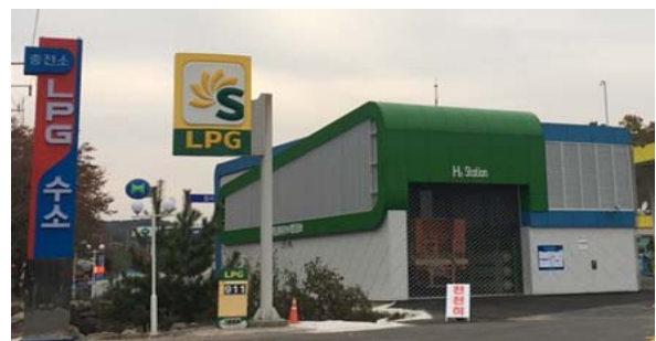
Fig. 1. LPG-Hydrogen Multi-Fueling Station
