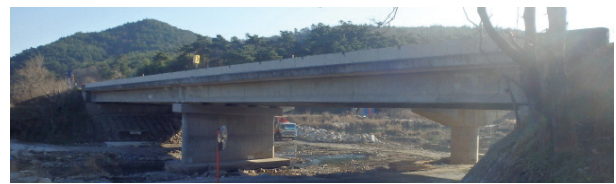
Photo 2 Overall View of Test Bridge
