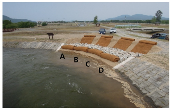
(b) Rolling Mat installation in bending channel
