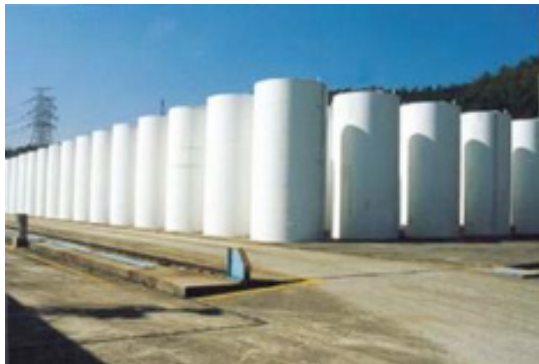
(a) Concrete Silo
