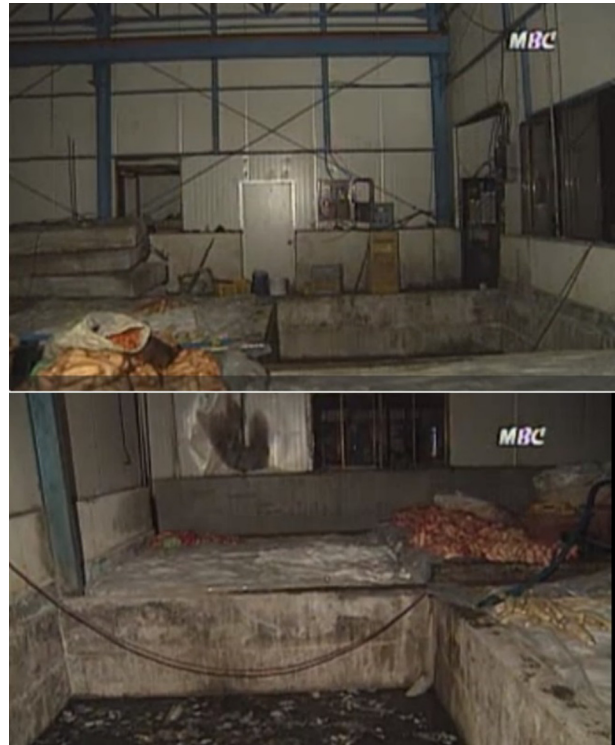
Figure 3. The danmuji(pickled radish) storage pit where 4 workers and a firefighter died by hydrogen sulfide asphyxiation(Nov. 15, 1996 in Sungju, Korea). [MBC News]
