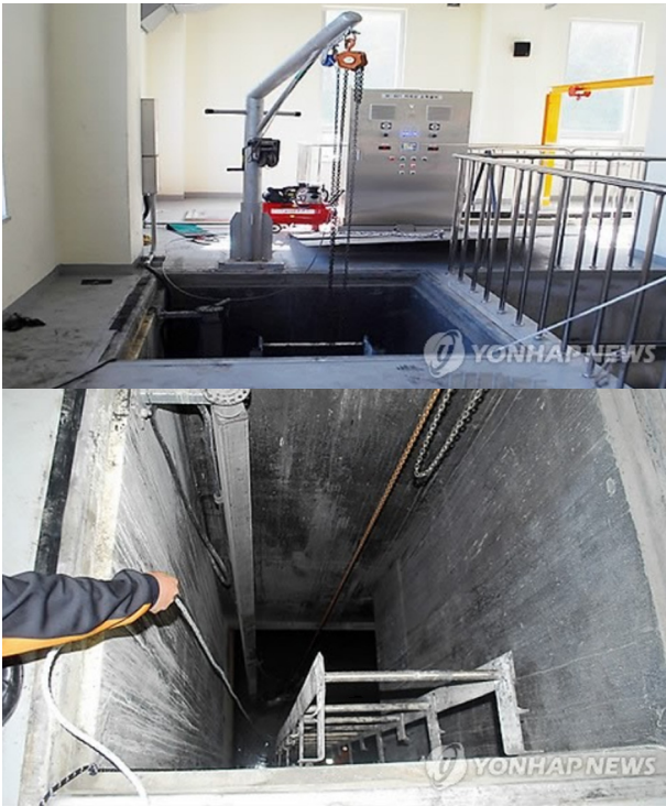
Figure 1. The wastewater treatment tank where a firefighter died in the line of duty (Oct. 30, 2012 in Ulsan, Korea) (Yonhap News photo).
