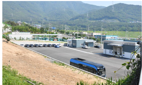
Fig. 1. View of Sung-ju hydrogen refueling station in Changwon
