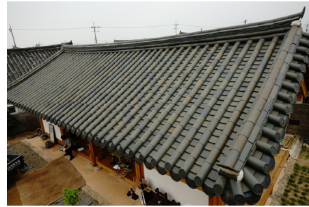
Fig. 15. Roof constructed by dry construction method with new Korean-style roof tiles
