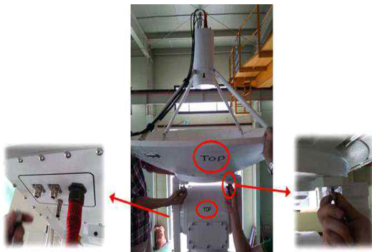
Fig. 9 Ground Antenna Installation Process
