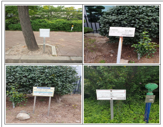
Fig. 7. Actual burial piping installation status.
