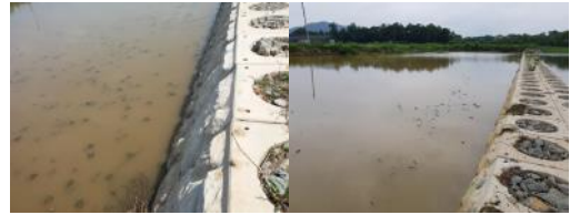
Fig. 2. Secondary dam for water purification
