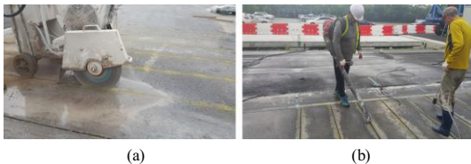
Fig. 7. Traffic sensor installation 1 st stage (a) Pavement cutting (b) cleaning operation
