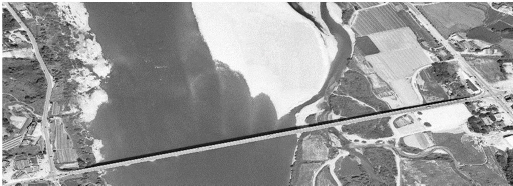
Figure 1. Entire Construction Site Photo
