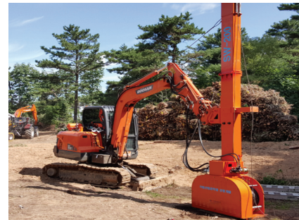
Figure 3. Tower-yarder based on excavator.
