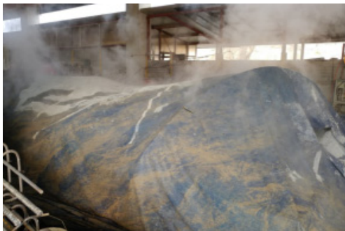
(e) Steam curing
