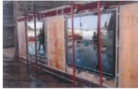
Fig. 5. Wind pressure test
