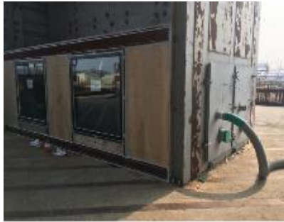
Fig. 3. Air Leakage test
