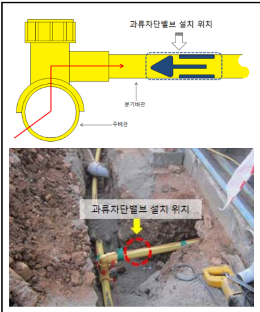
Fig. 3. Installation spot in LPG pipeline
