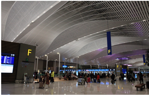
Fig. 1. The slat structure used on the ceiling of the second terminal of the Incheon international airport.
