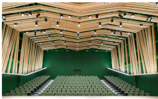
Fig. 2. An example of slat ceiling used in a concert hall (William M. Lowman Concert Hall, California, USA). [2]
