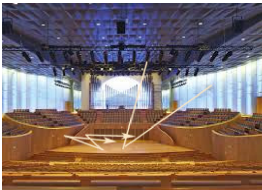
(b) Lack of early reflections in vineyard stage Fig. 3. Stages in shoebox/vineyard concert hall.
