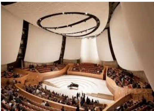
Fig. 4. Stage reflector on the wall.
