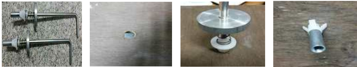
Fig. 4 The Buoyancy Prevent Device of Hollow Core Materials and Fixing Method
