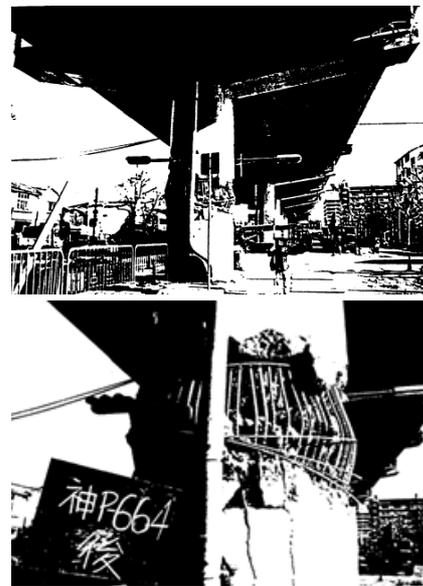
Fig. 3. Representative Observed Damage Pattern of Pier P664 (Elnashai et al., 1995)
