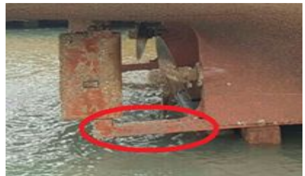
Fig. 8. Structure near the propeller underneath.
